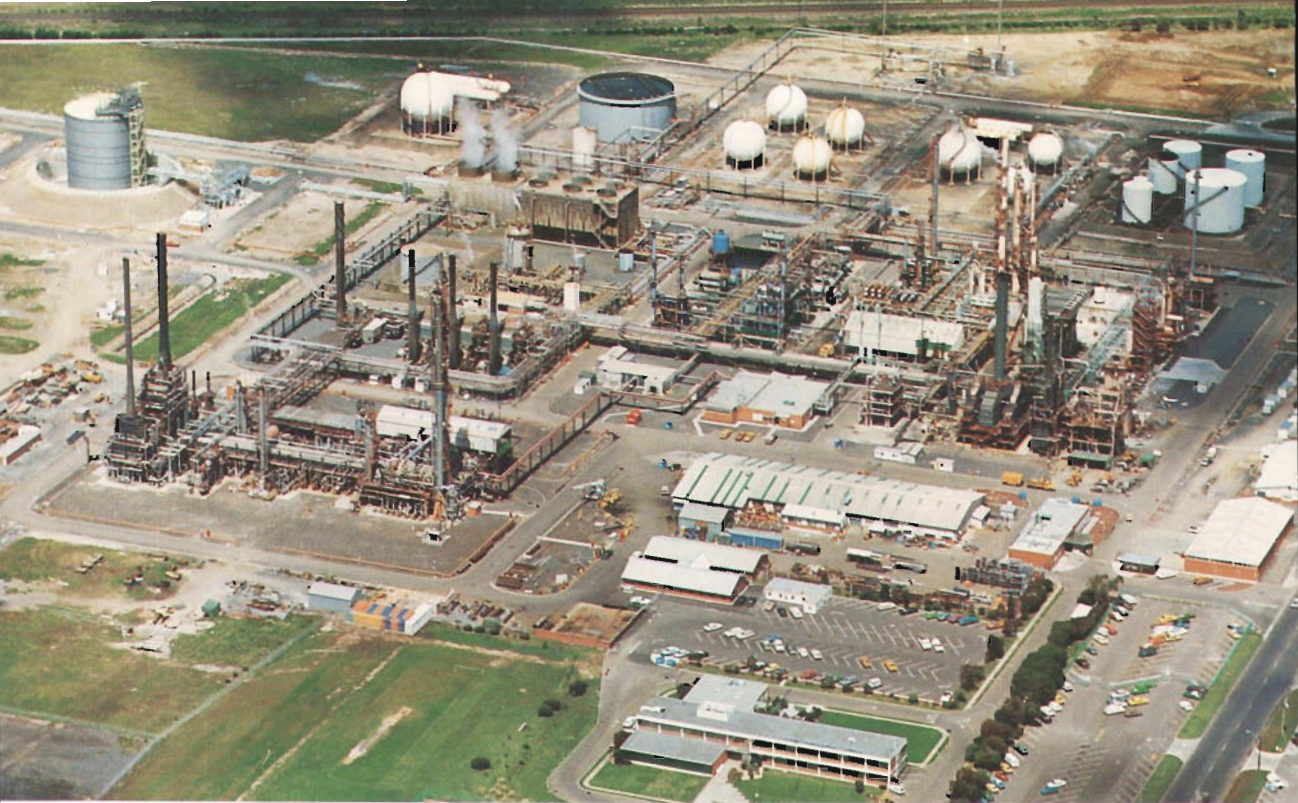
The plant of Altona Petrochemical Company which is engaged in chemical, synthetic rubber, and plastic production.
